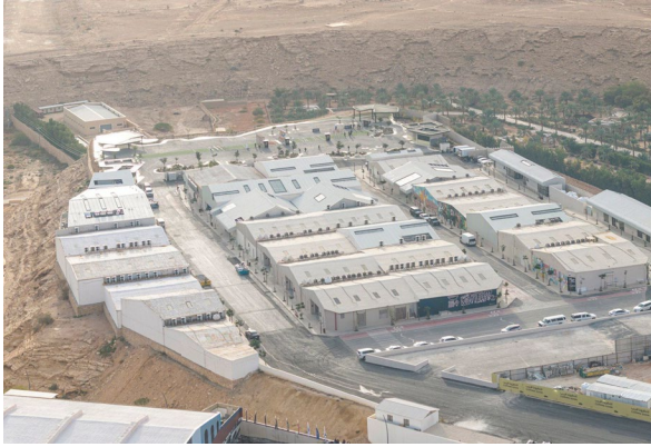
Figure 1. Aerial view of JAX. (Laurian Ghinitoiu, via ArchDaily, 2024)
