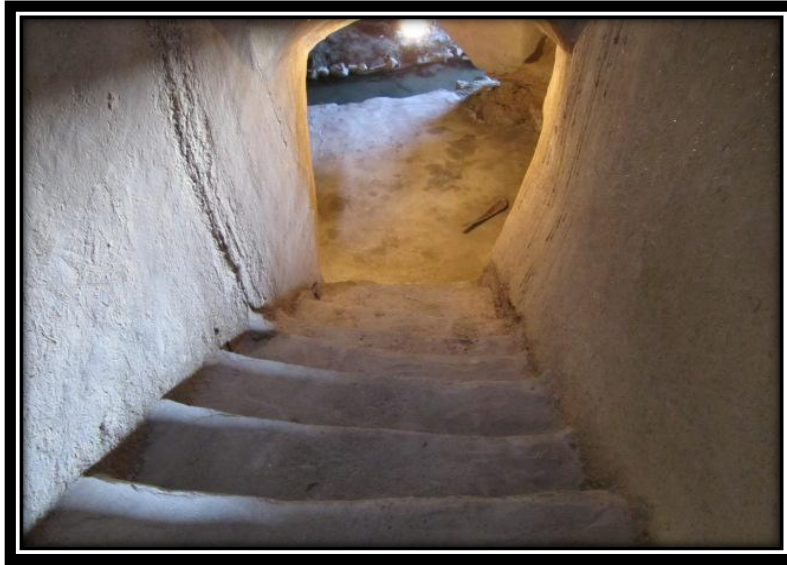
Fig. 2 The Payab of Bayazeh Qanat from inside a house in the village of Bayazeh
